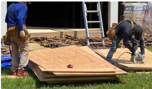
Cutting plywood to fit the ridge area.
