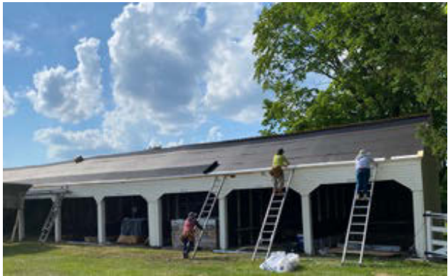
Unrolling the Cedar Breather 1/4" mesh to let the shakes breathe.
