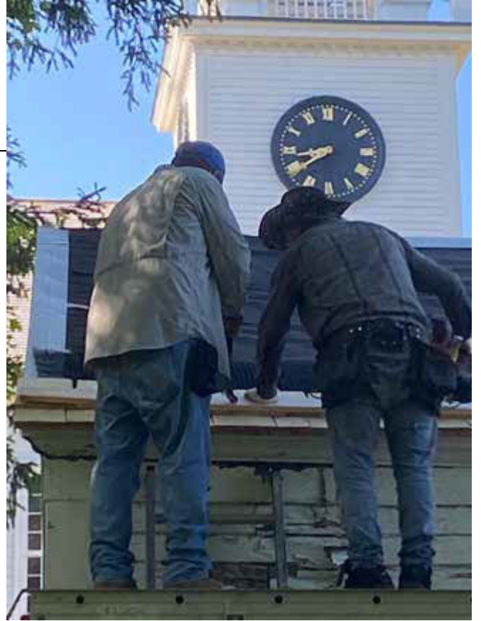
Foreman Harry St. Lawrence and crew member use a long alignment board to align the first row of shakes at the base of the back roof.
