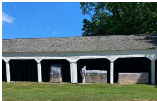
7:30 a.m. 6/22/20 Ken inspects supplies. At 8:00 a.m., a Guyer & Sons Roofing veteran crew of 7 men and a woman began working.
