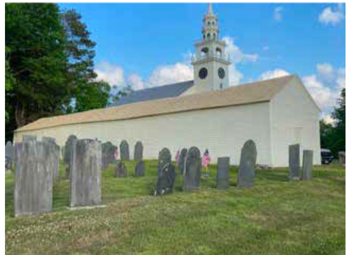
Back side shingled by end of Day 2; front is still felt. Meetinghouse's 2017 yellow cedar has weathered to gray.
