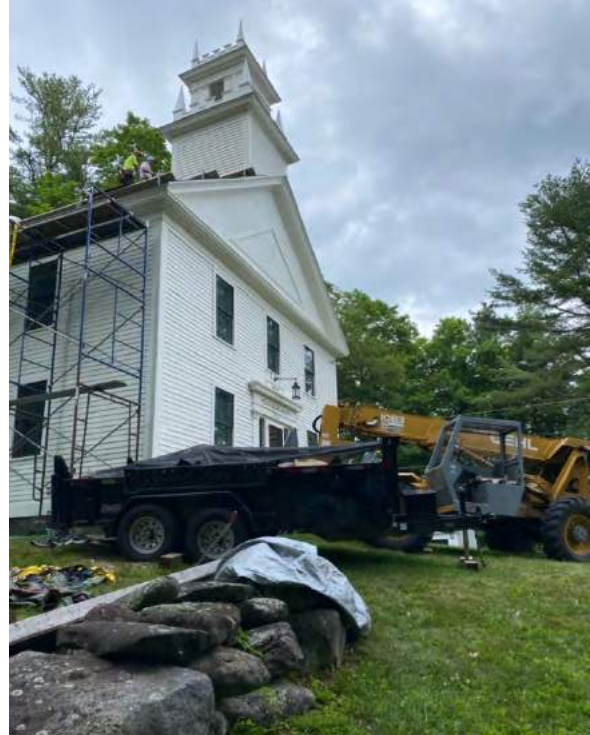
Heavy equipment including a 40' lift was necessary to do the re-roofing.
